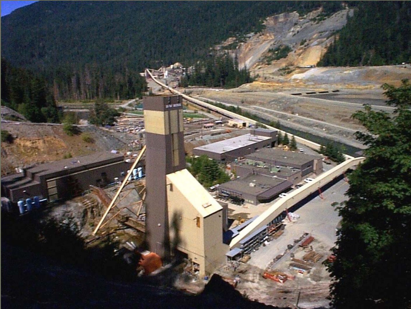
1 – This is an aerial view of the head frame at Myra Falls Mine in Strathcona Park on Vancouver Island.
