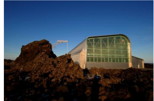
Alterra's Power Plant in Reykjanes, Iceland
