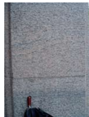
Figure 19 – Panels of banded gneiss at the base of The Centre. (Umbrella handle for scale.)
