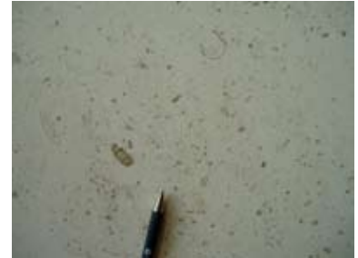
Figure 4 – Pale yellow limestone with scattered marine fossils, foyer walls at 250 Howe Street.
