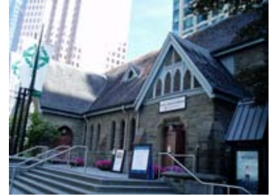
Figure 29 – Century plus-old Christ Church Cathedral constructed from sandstone.
