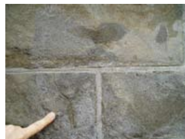
Figure 12 – Gabriola Sandstone blocks make up the wall around and foundation of Holy Rosary Cathedral.
