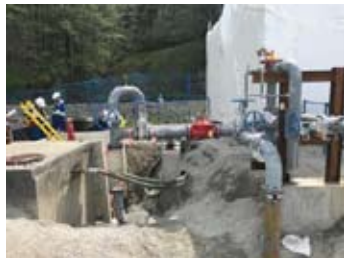
April 2018 – new firewater line
