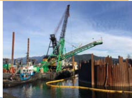
Circular Sheet Pile Cells – for Cofferdam, September 2019
