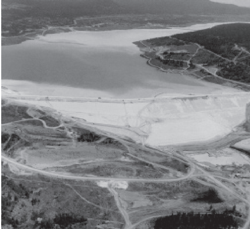
Tailings Pond at Highland Valley Copper Mine near Logan Lake, BC
