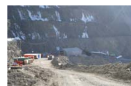
Portal into the underground at the bottom of the Afton pit.
