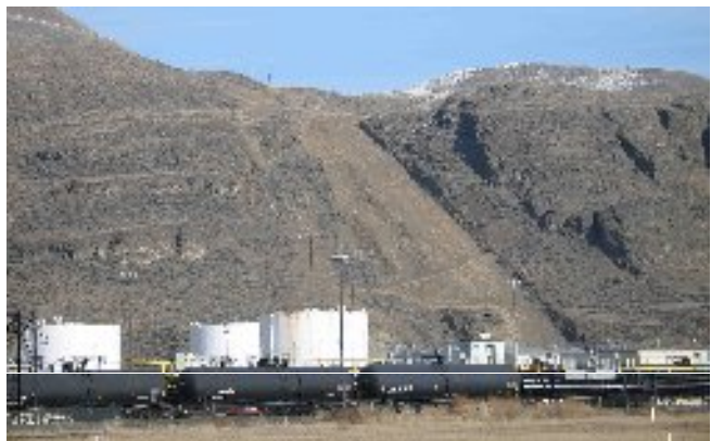
Figure 50. (Below) The smoothed and revegetated scar marks the buried route of the Trans Mountain Pipeline up the valley slope north of the petroleum depot and airport. The pipeline transports gasoline and diesel, each in separate batches, over 1000 kilometres from refineries in Edmonton via Kamloops to Vancouver and Washington State. The 60 cm diameter pipeline is owned by Kinder Morgan Ltd. and can transport over to 250,000 barrels of oil per day. (Photo by R.Turner)
