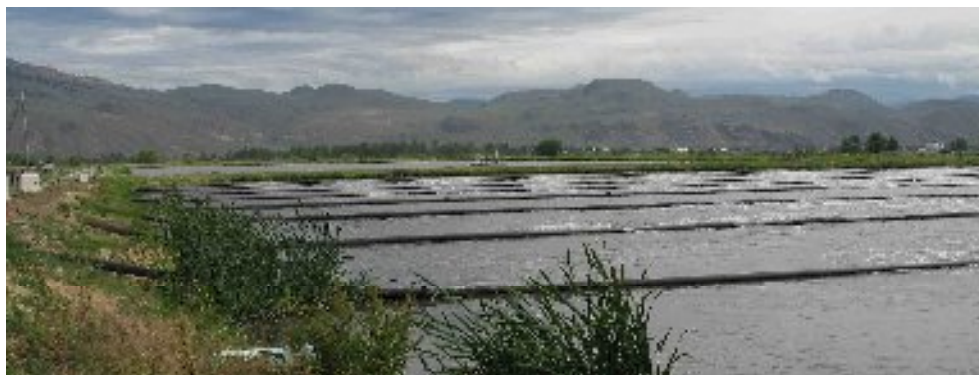
Figure 56. Bubblers within the secondary treatment lagoon mix oxygen into the wastewater. This oxygen is essential to sustain bacteria that feed on and digest the organic matter, converting organic compounds to non-harmful products. Abundant green algae on the surface and shoreline plants reflect the nutrient-rich nature of the waste water. (Photo by R..Turner)
