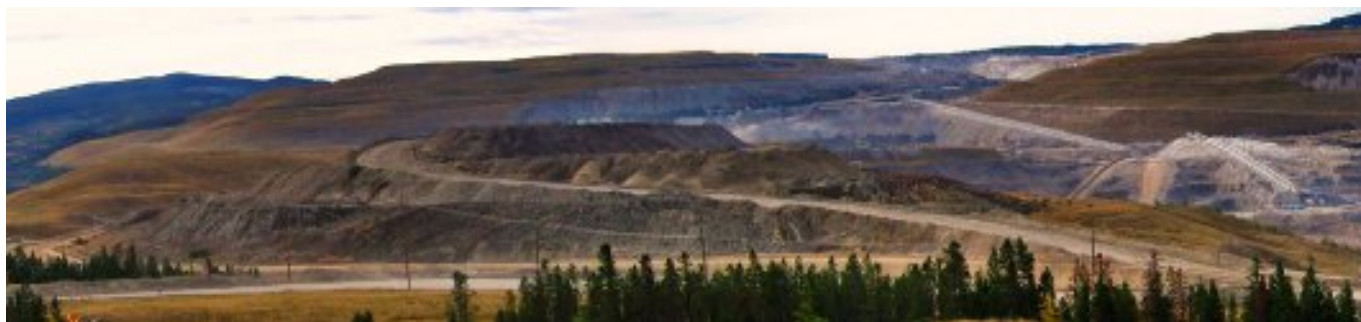
Figure 44. A view of the active mining area and surrounding reclaimed mine dumps. The reclaimed mine dumps are golden brown grasslands that have been smoothed, covered with soil, and planted with grasses. The conveyor belt is the white diagonal line and transports ore from the mine pit (lower right) to the mill (centre and hidden behind active rock waste dumps). (Photo by R. Anderson)
