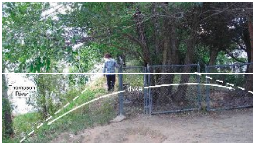
Figure 27. The integrity of this dyke on the North Shore along the Thompson River may be compromised by the trees that grow on it. Trees can weaken a dyke; when tree roots die, they leave behind small tunnels that can allow water to flow through the dyke during a flood. Such small water flows can lead to larger failure of the dyke. (Photo by R.Turner)
