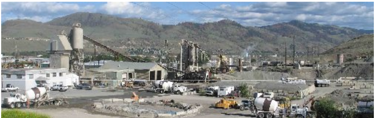
Figure 47. (Above) A redi-mix concrete and asphalt plant, and gravel pit along Yellowhead Highway 5 at Paul Lake Road. Sand and gravel deposits are sorted by screening into separate piles of gravel and sand, and used in the production of concrete. (Below) Sand,
